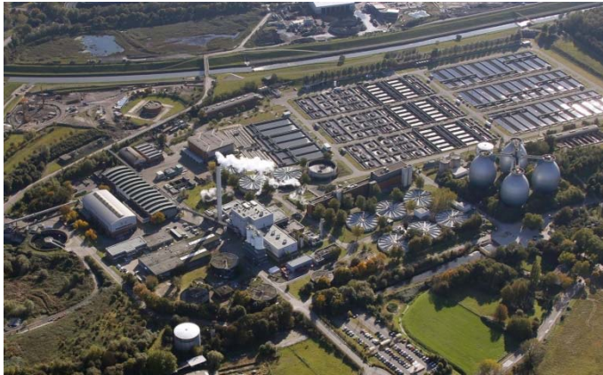
Figure 66: WWTP in Bottrop in the Emscher area, one of the largest WWTPs in Germany, with an electricity consumption of 40 M kWh per year.
